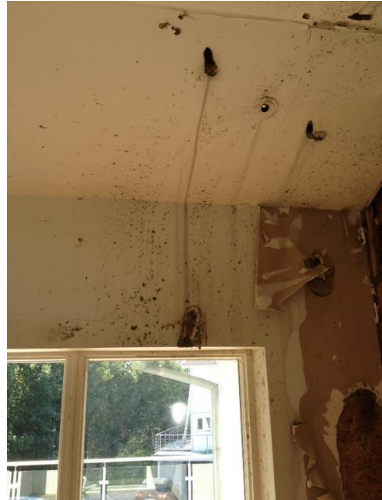
Damage caused by the cutting extinguisher
